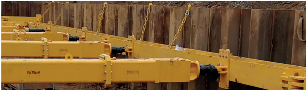
Fig. 1: example of assembly of hanging chains
